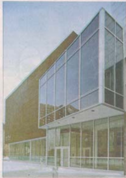
JOEL EDWARDS • jedwards@startribune.com Shiny glass contrasts with rust-coated Co-Ten steel at the west entrance to MacPhail Center for Music.
